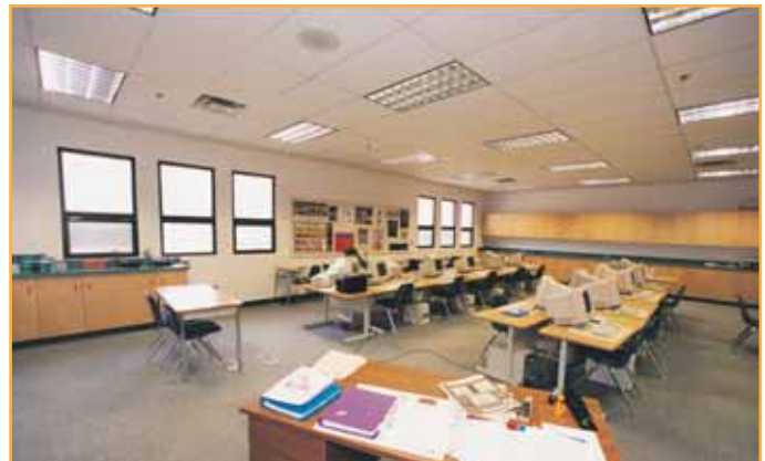
Radiant ceilings frees up wall space for cabinets.
