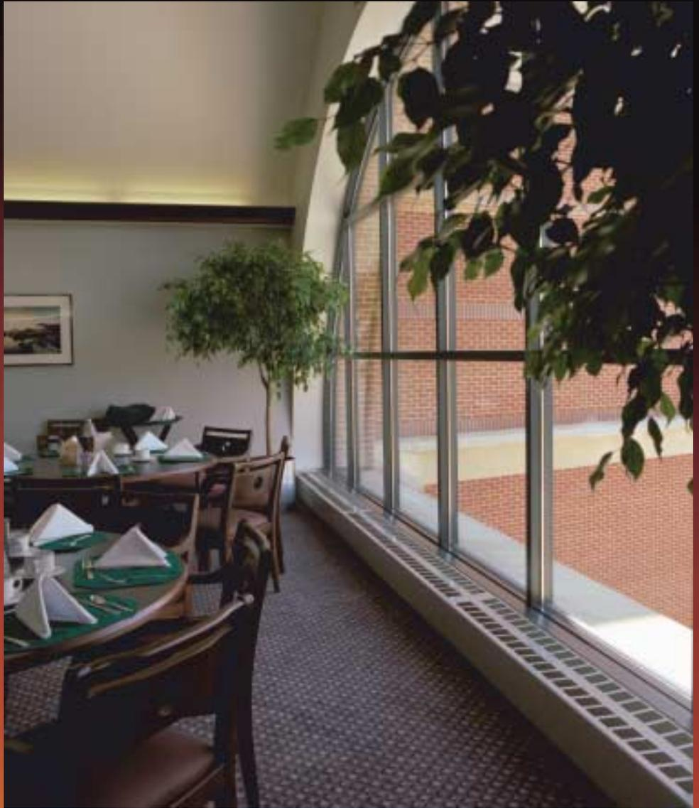
Hydronic Finned-Tube Radiation
